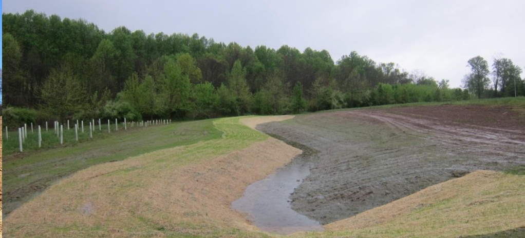
Level lip spreader after construction
