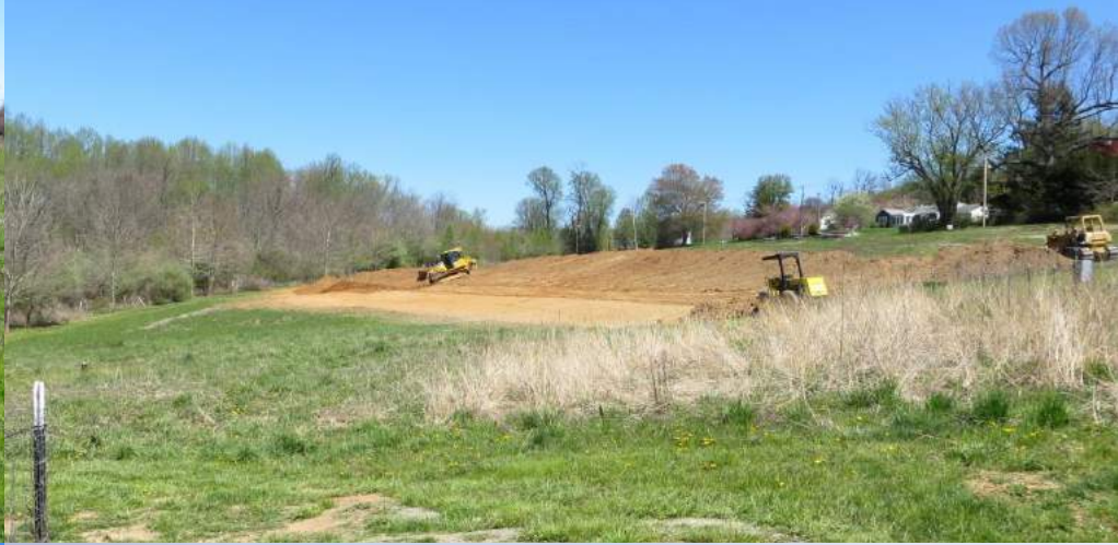
Level lip spreader after construction
