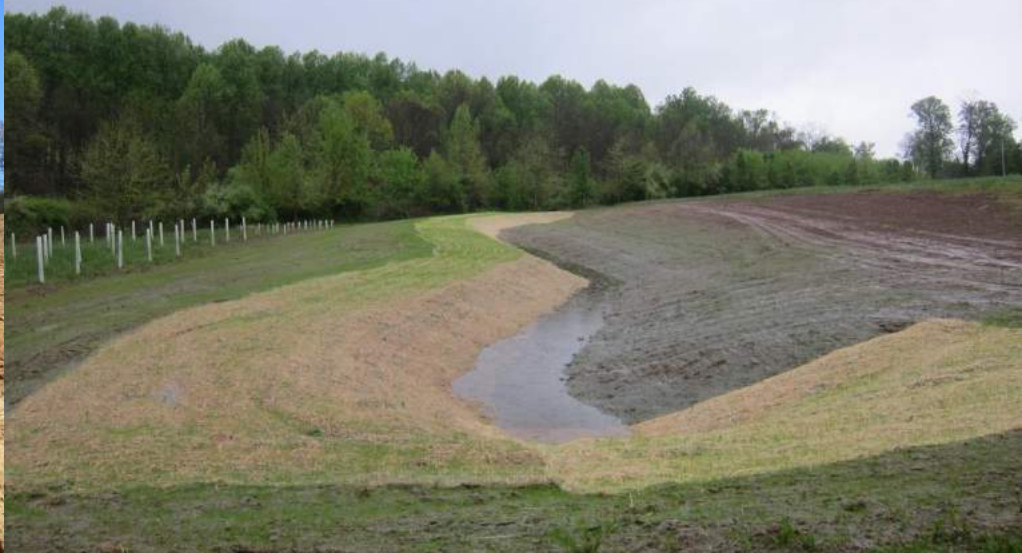
Level lip spreader after construction
