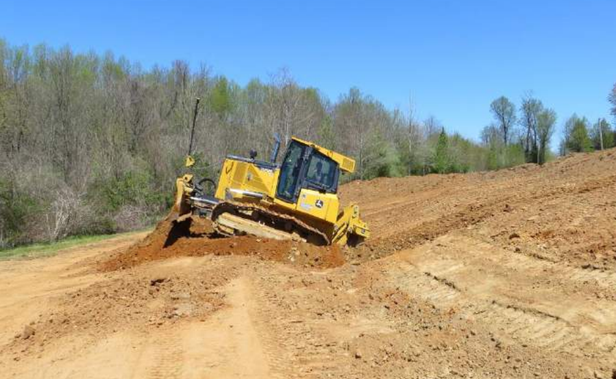
Level-lip spreader during construction
