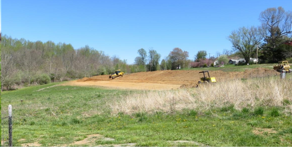
Level-lip spreader during construction
