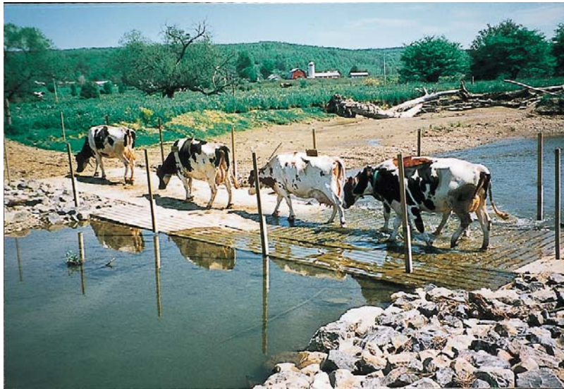
Figure 11. Stabilized stream crossing.
